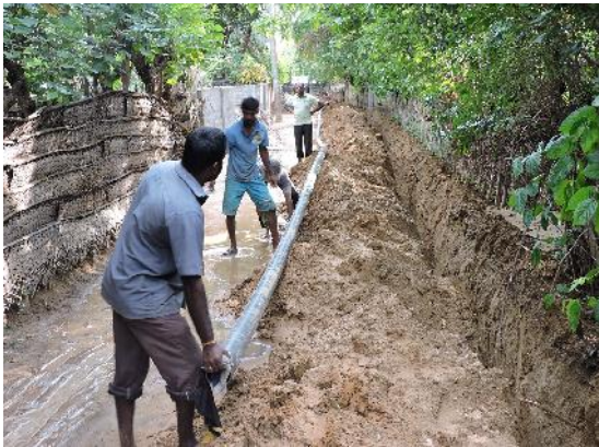
WASH CBO monitor the pipe laying work
