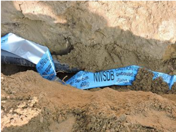
NWSDDB's technical support for pipe laying
