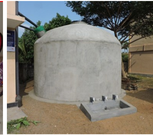
A 30,000 litre rainwater harvesting system constructed in schools.
